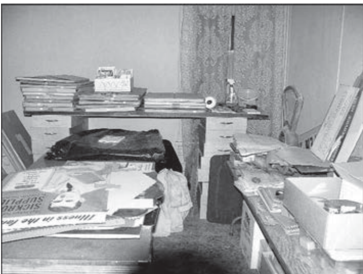
These are the second floor rooms that will be renovated. Walls must be removed, loose plaster removed and replaced with drywall, 9' insulated dropped ceilings hung, flooring overlaid and tiled, and furnace/air-conditioning installed.
