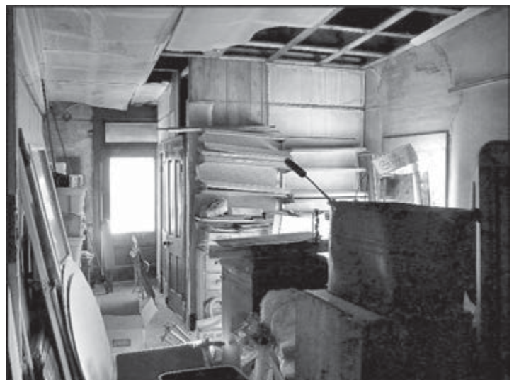
These are the second floor rooms that will be renovated. Walls must be removed, loose plaster removed and replaced with drywall, 9' insulated dropped ceilings hung, flooring overlaid and tiled, and furnace/air-conditioning installed.
