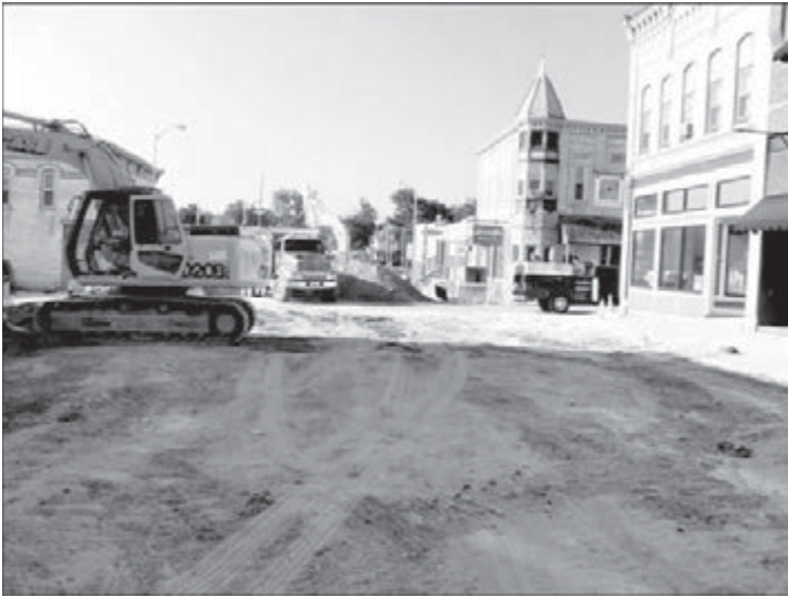
Monticello's Main St. construction before the October 2010 completion. The museum's under-sidewalk coal bin had to be filled in to accommodate the new sidewalks.
