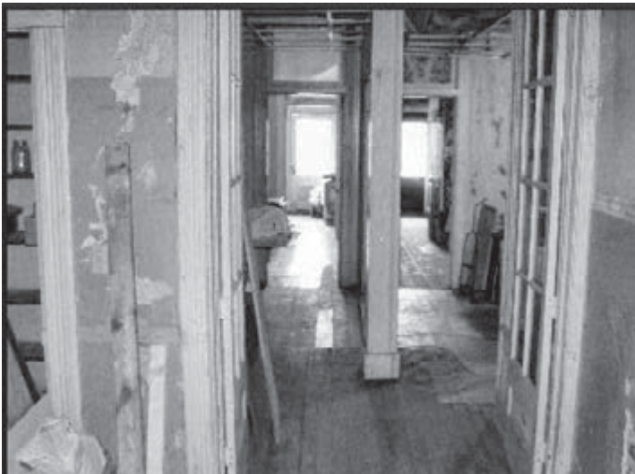
These are the second floor rooms that will be renovated. Walls must be removed, loose plaster removed and replaced with drywall, 9' insulated dropped ceilings hung, flooring overlaid and tiled, and furnace/air-conditioning installed.
