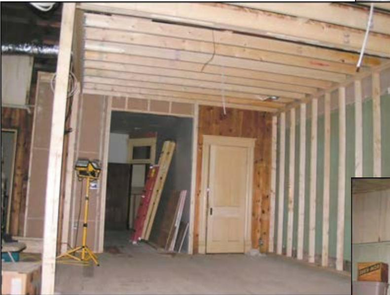
The construction on the north side of the floor is done, furnace and ductwork are installed and the electrical wiring is roughed in. Insulation and drywalling will be done soon,
